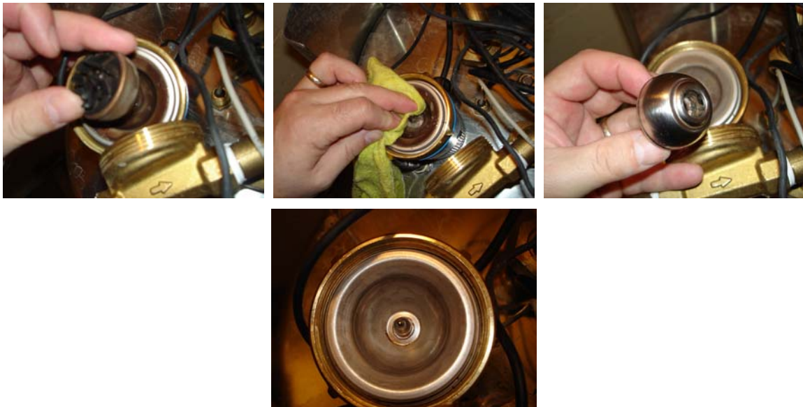
Take out the impeller wheel and clean this thoroughly, along with the pump housing.
